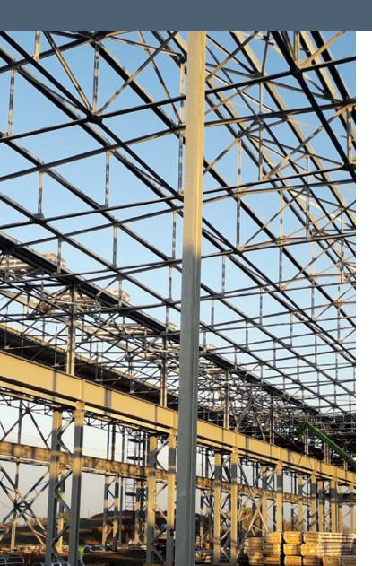
One of **Bertoli Costruzioni** 's added values is a state-of-the-art construction system, which drastically reduces installation time and eliminates long production downtimes. Prefabrication is carried out in-house or in an area made available to the client. The blocks follow a precise and functional identification system.
